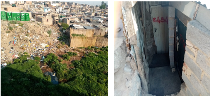
Figure 3: Living Conditions in Stjwetla. Source: Authors' construct (2020)
