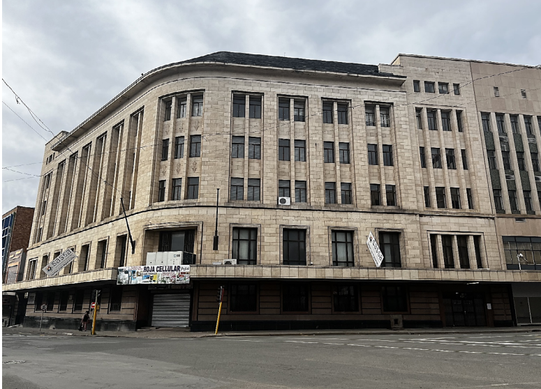
Figure 16: Historical Building in Kimberley. Source: Researchers' (2022) own photograph
