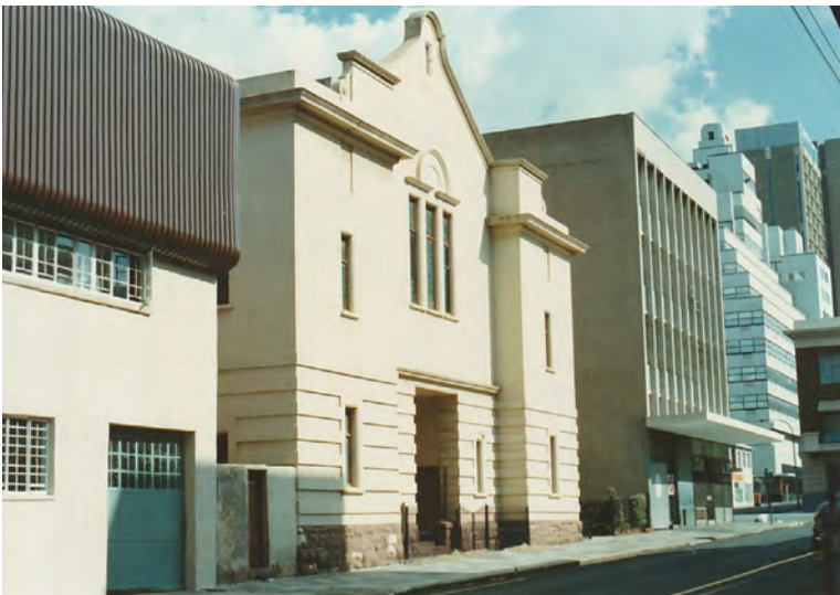
Main entrance of Albert Street Methodist Church. Taken in late 1990's.
