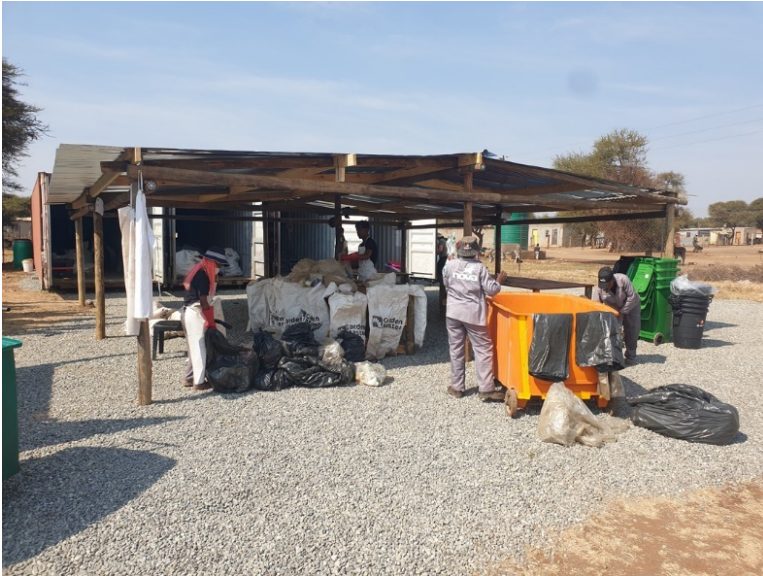
Figure 15: Local waste sorting facility
