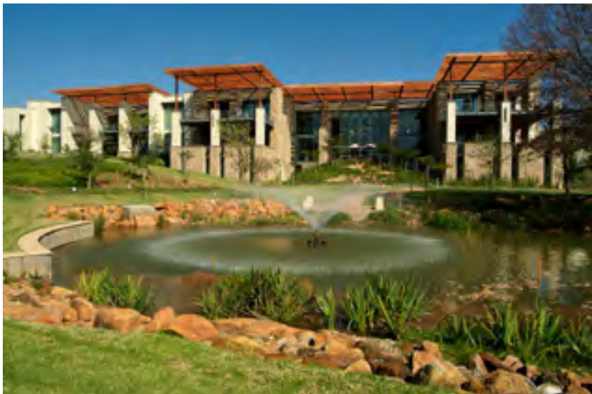
Above right: Vodacom Campus, Midrand, 1998. Right: Vodacom SSIC, Midrand Photographer: Barry Goldman Left: Standard Bank Global Leadership Centre, Morningside, 2007. GLH Archive.
