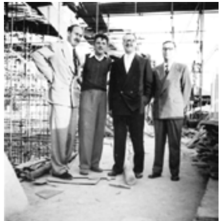
Above: Manfred Hermer with a model of the Durban Ice Drome, and Hermer (left) and team on site during construction, 1955. Left: Durban Ice Drome 1955, GLH Archive.
