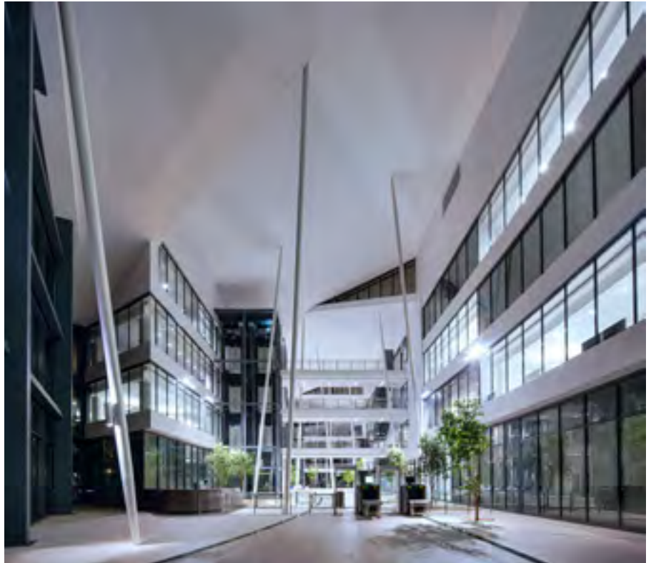
Left: main entrance. Right: internal atrium. Photographer: Barry Goldman.
