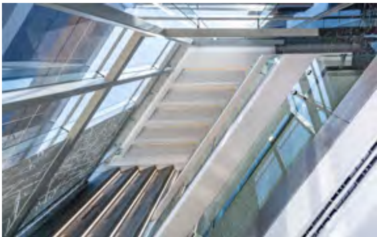
Far left: 2 Pybus Road, 2019. Left: 2 Pybus Road, atrium ceiling Source: Infrastructure Photos.
